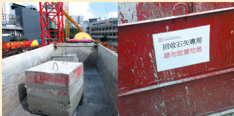
▲ Recycling of residual concrete
