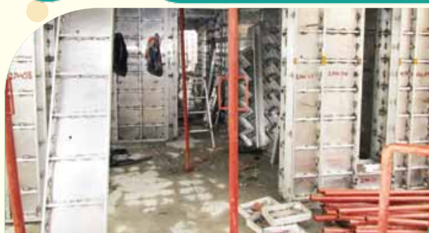
Use aluminium formwork to reduce use of timber
