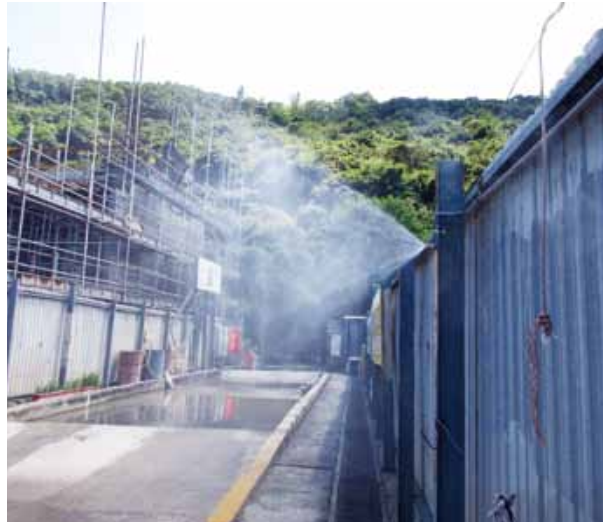
Collect surface runoff and gray water for vehicle washing and dust suppression
