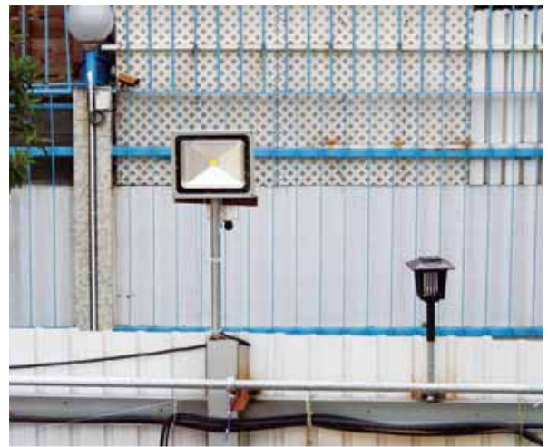
Replacement of LED floodlight
